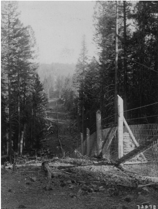
Figure 1. The coyote-proof pasture fence, Wallowa National Forest, 1907, shortly after construction. Trees were cleared for 10 feet on either side of the fence to prevent wild cats from leaping over from overhanging branches. One strand of barbed wire was stretched along the ground surface to discourage predators from digging underneath. Photo courtesy of the National Archives, College Park, MD.
